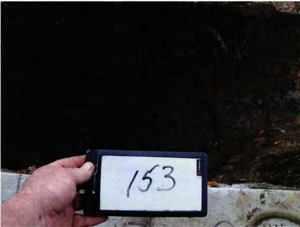
Picture 2: UST 153LaurelBB excavation.
